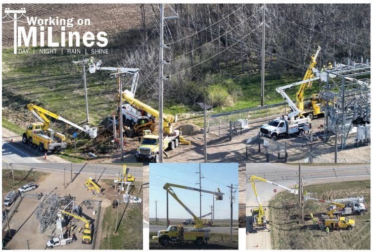
MiEnergy crews, along with two Dairyland employees, are pictured removing all overhead lines exiting the Saratoga substation and converting them to underground electric feeders. This is the last of four substations including Alta Vista, Lime Springs and Schley to complete the same process in Iowa. Crews changed 69-kV insulators and failing fuse brackets. They also removed other deteriorating equipment to improve system reliability
