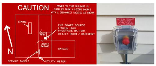
**E-Stop-** Emergency stops were installed at all four sites. Three of the four were installed outside of the house with one being near the doorway that enters the utility room. The E-stop allows anyone to quickly turn off the battery unit without having to open the battery unit or entering the room and using the utility disconnect.
