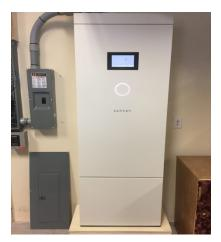
Pulsing White: Normal operation Pulsing Green: Off-grid operation Pulsing Orange: No Internet connection Pulsing Yellow: Firmware/System Update Solid Red: Error
