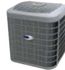
The split system is a version of ASHP that functions with indoor and outdoor components, transferring heat from the house to be evaporated outdoors in the summer, and transferring warmth from the outdoors to heat the house during the heating season.
