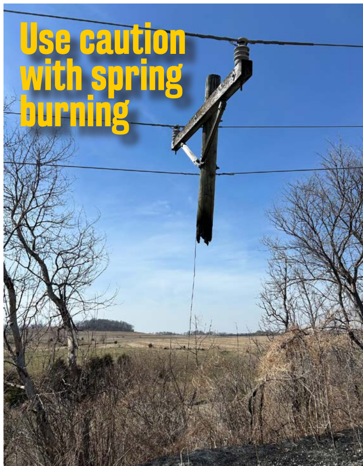
This is a photo of a MiEnergy pole taken the week of March 23. It is a good reminder to use caution when burning near power lines. Beyond power poles, there can be cabinets, transformers for underground service and guy wires hidden in the tall grass or other overgrown vegetation. If these burns are not managed safely, they can cause property damage, power outages, injury, and even death. Burning a power pole or other electrical equipment could cause a widespread power outage and be costly for the individual responsible for the fire.
